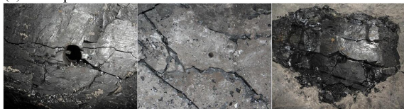
(b) Concrete specimen
