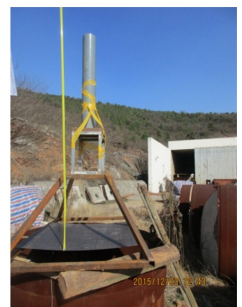
图6 侵入实验现场布置
