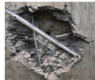
(b) Back of the wall
