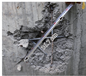
(b) Back of the wall
